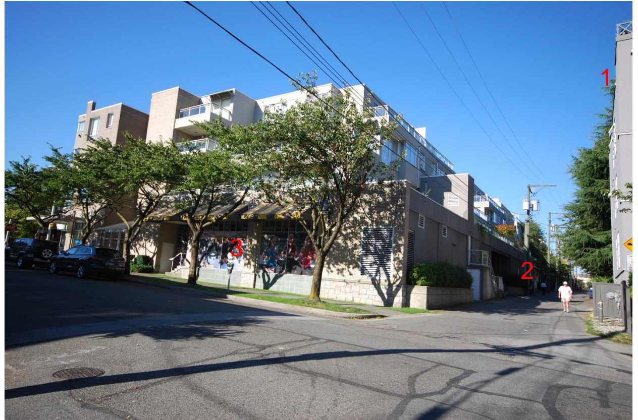
View of the Capers Building from Yew Street, showing the integration of the large building into the neighbourhood context via a back lane.
