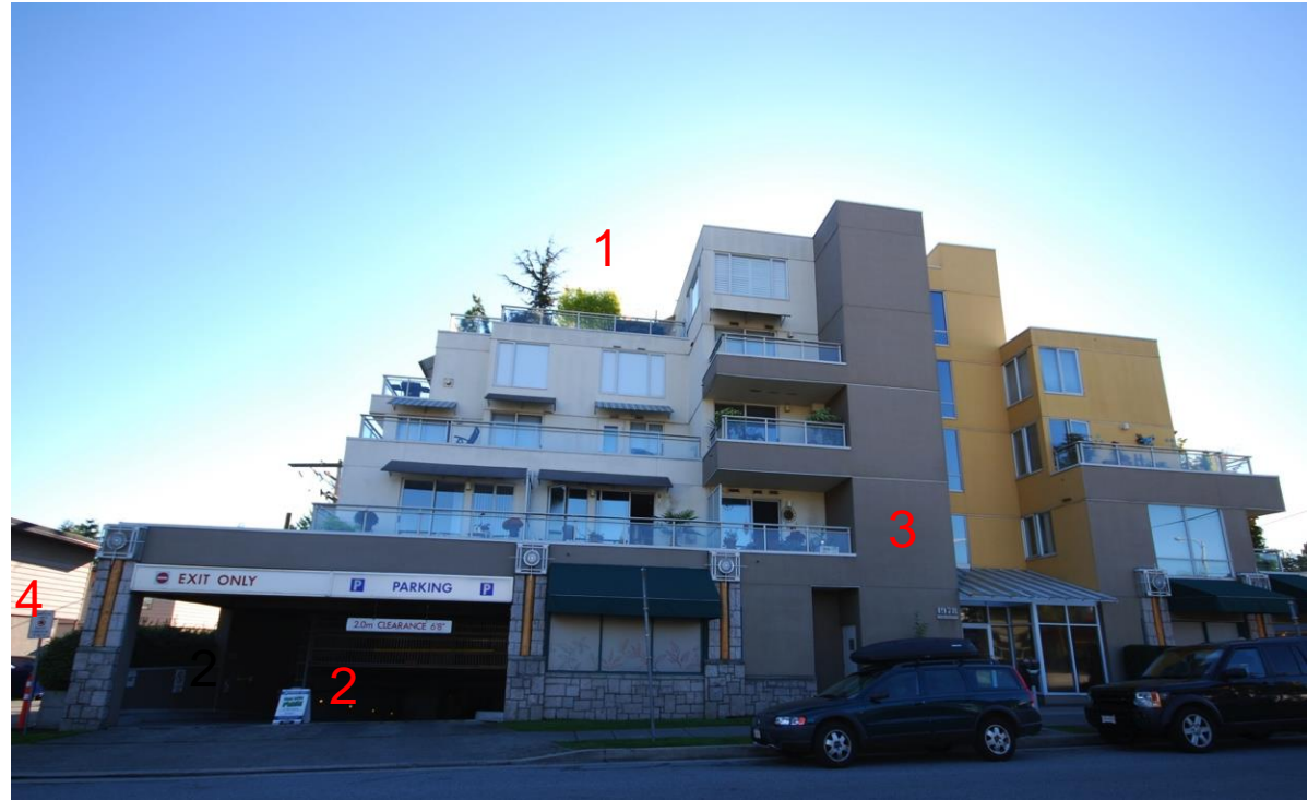
The side street at the western end.
