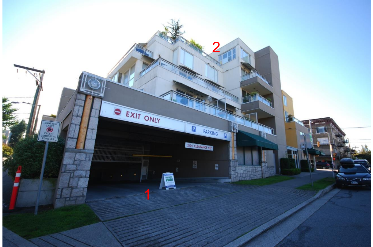
View of the western end of the building, showing the entrance to the basement parking.
