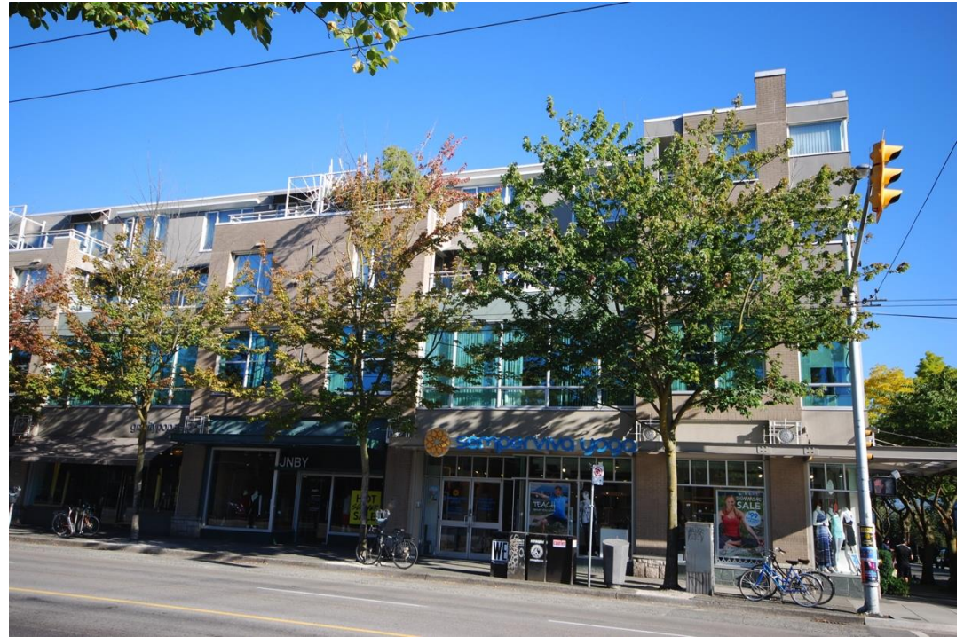
View of the four storey building with retail on the ground floor, office space on the 1 st floor, and residential above.
