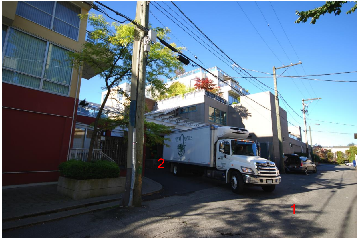
View west along the back service lane showing one of two service docks along its length.
